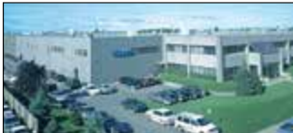
Montreal, Canada Velan Inc., Plant 2 and 7
