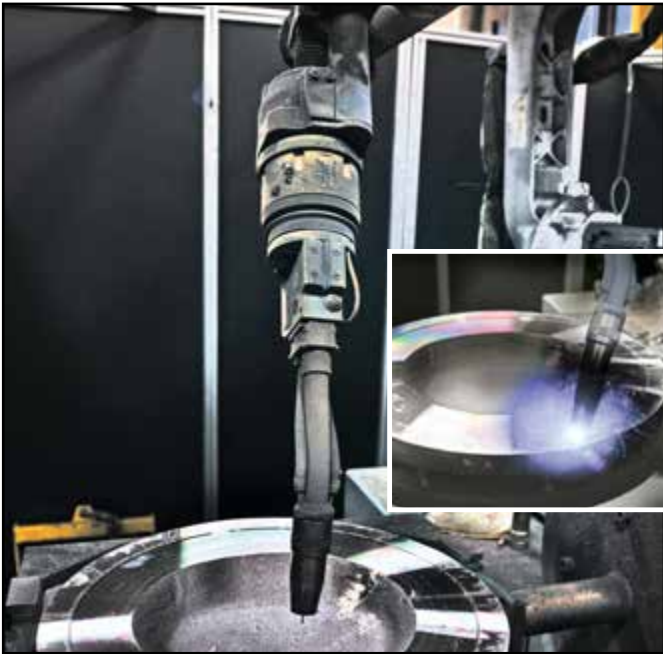
Automatic plasma arc hardfacing equipment of a wedge using a robotic arm.
