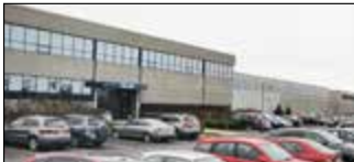
Montreal, Canada Velan Inc., Plant 5
