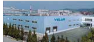
Ansan City, South Korea Velan Ltd., Plant 2
