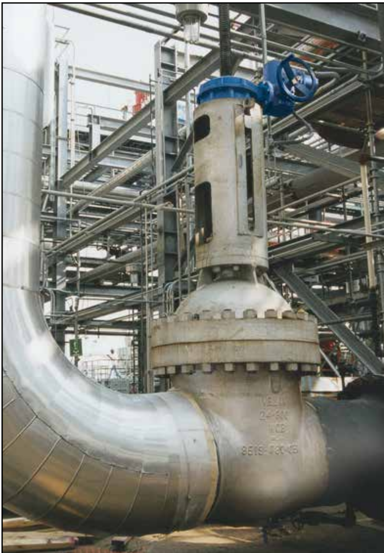
Carbon steel gate valve, ASME Class 600 used for boiler feed water installation at a hydrogen plant in Texas.
