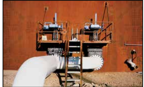
Cast steel valve installation at an oil refinery.
