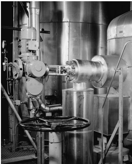
H.P. preheater in a nuclear power station equipped with a condensate drain control valve type ZK 29
